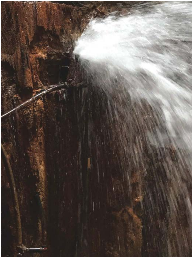
Fig. 2: Major water penetration points were blasting masses of water 12 in (300 mm) wide across the 23 ft (7 m) diameter of the shaft. The extreme pressure of the water was causing damage to the shaft structure and made the repair a very dangerous project.
