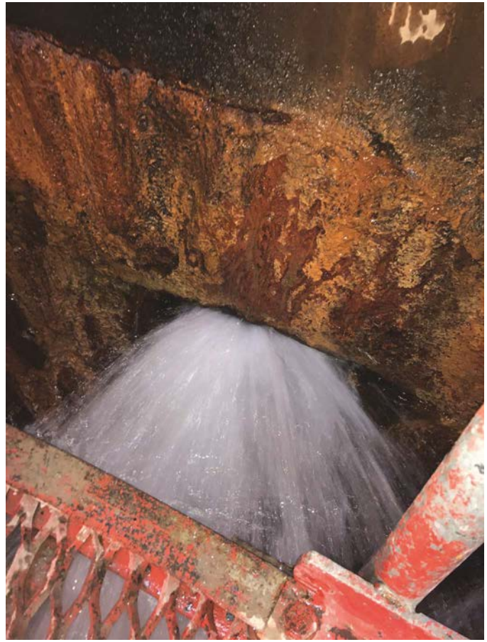
Fig. 2: Major water penetration points were blasting masses of water 12 in (300 mm) wide across the 23 ft (7 m) diameter of the shaft. The extreme pressure of the water was causing damage to the shaft structure and made the repair a very dangerous project.
