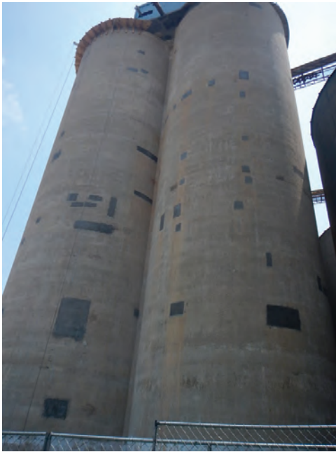
Miscellaneous repairs, West Elevation; note formwork at roof slab overhang
