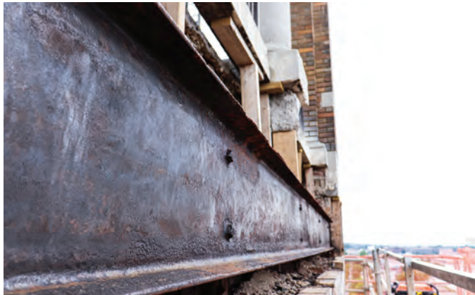
Fig. 6: Steel beams exposed below tower lookout
