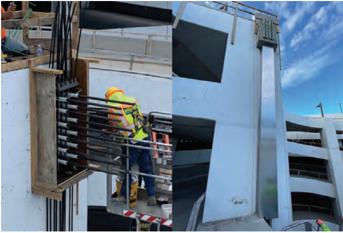
Fig. 11: One new anchor block for the vertical external post-tensioning system at the top of the column
