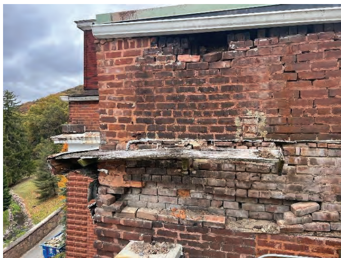
Main kitchen wall failure after removing the existing copper cornices. The entire length of the wall would require replacement
