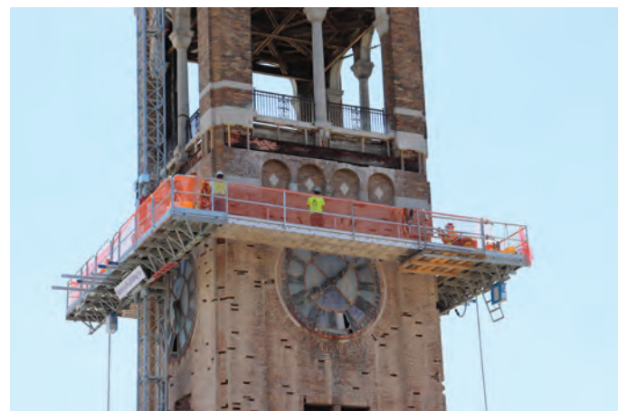
Fig. 4: Bridge pick to allow mast climber to reach ground on at least one side
