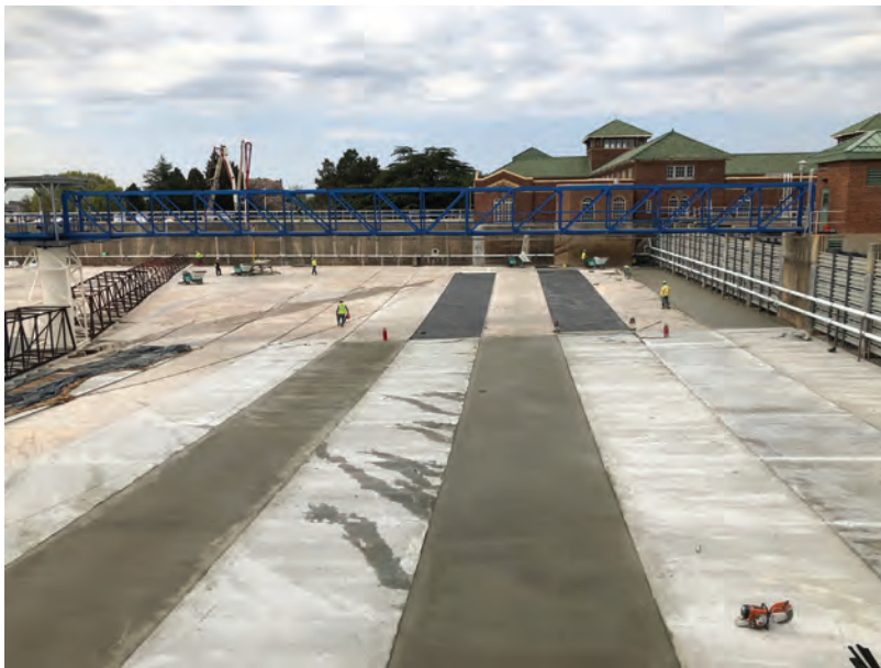
Concrete overlay being poured in strips
