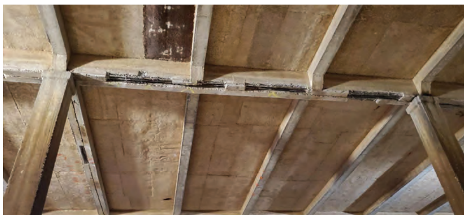
The visible spalled concrete beams exhibit significant rebar corrosion
