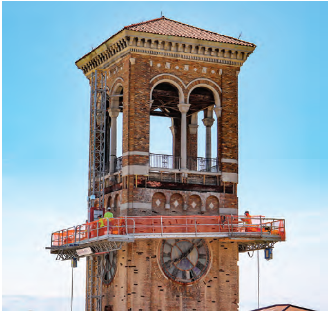
Fig. 5: Brick/stone removed to access "shelf angle repairs"
