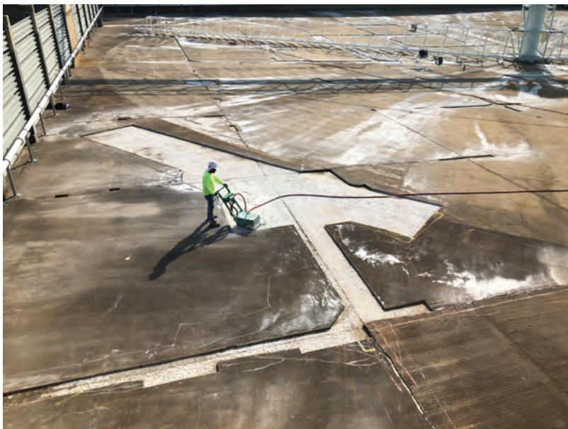
Saw cutting of the edges for concrete repair
