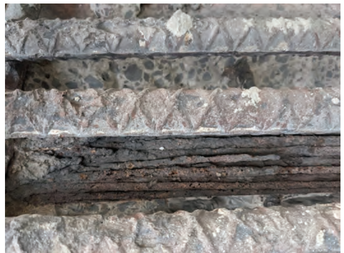
Fig. 3: Fractured and heavily corroded girder tendon exposed in a concrete repair opening
