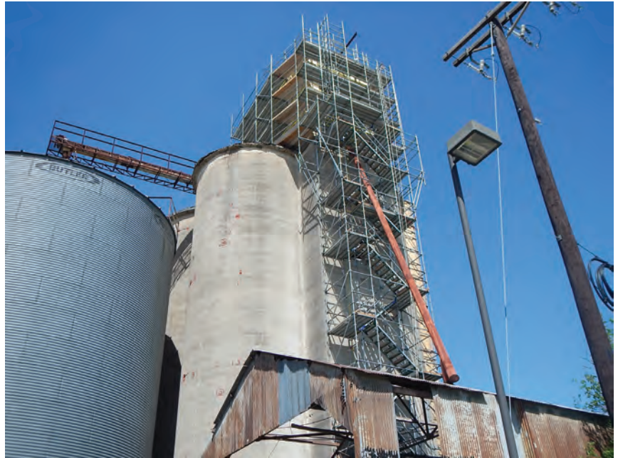
Tagging of repairs and demolition of doghouse in progress
