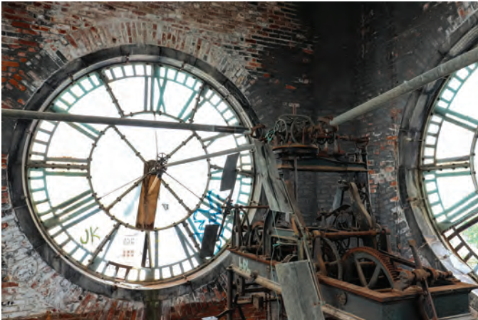
Fig. 2: Clock tower glass/mechanicals prior to restoration
