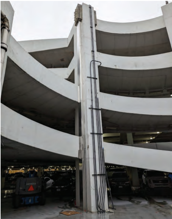
Fig. 14: Finished EPT column repair with stainless steel cover protection against UV degradation
