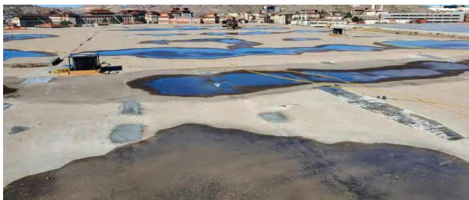
Water-ponding on the tank roof after rainfall
