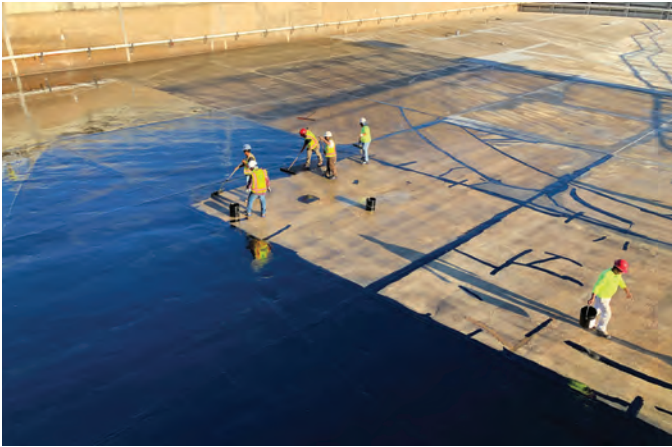
Application of the waterproofing coating
