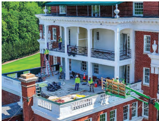
Tower terraces after structural repairs were completed and parapets reconstructed with restored balustrades. Installation of new balcony guard railings in progress
