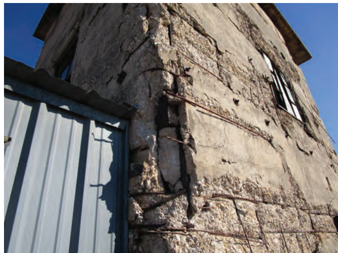
The doghouse deterioration was so extensive that it had to be removed
