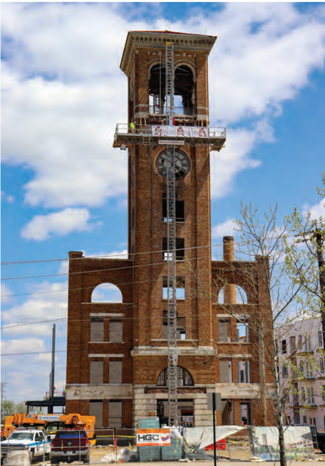
Fig. 3: Four-sided mast climber on tower
