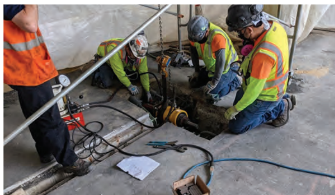
Fig. 4: Girder PT restressing
