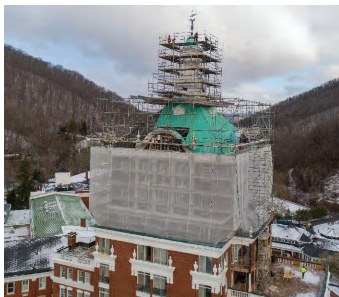
Scaffolding system at the main tower with copper roof restoration and façade repairs in progress
