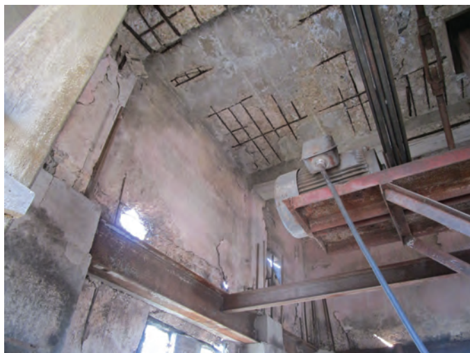
Doghouse interior; note deteriorated concrete, added steel framing, and equipment that required removal
