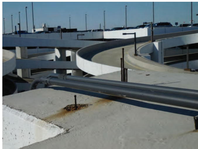
Fig. 9: Failed post-tensioning wires erupted from top of a helical ramp column
