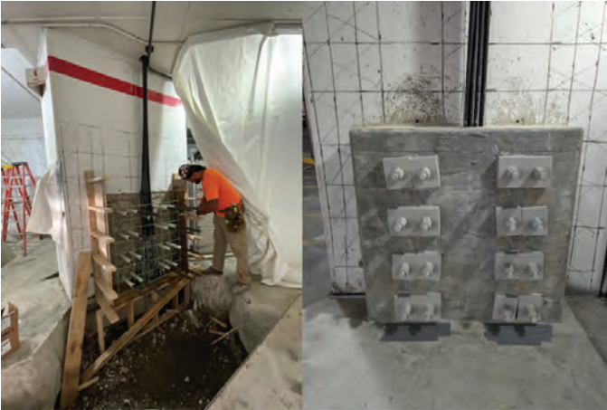
Fig. 12: One new anchor block for the vertical external post-tensioning system at the base of the column
