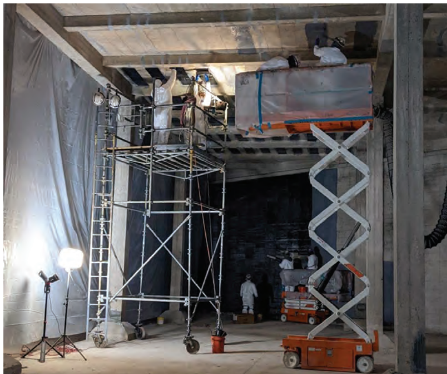
Sectioned areas of the tank heated while FRP is being installed
