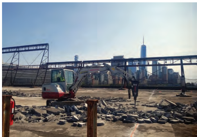
Demolition of concrete slab
