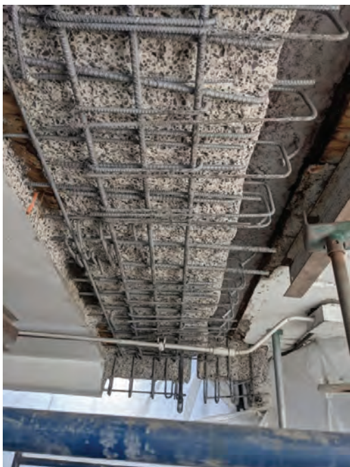
Fig. 8: Repair of deterioration of the underside of the ramp slab at the joint between the ramp and the parking deck
