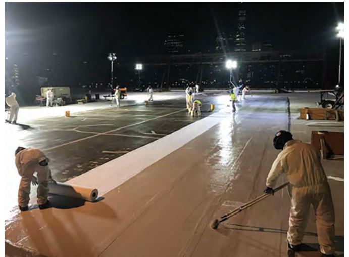
Installation of new waterproofing system
