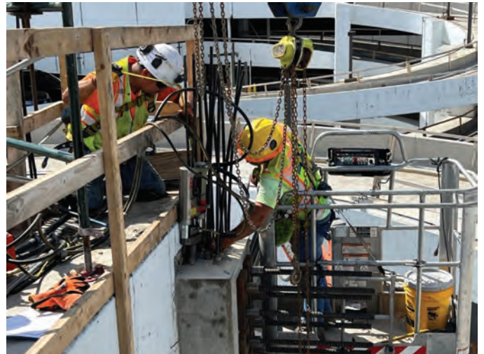
Fig. 13: Stressing of the vertical external post-tensioning tendons strengthening the cantilevered column
