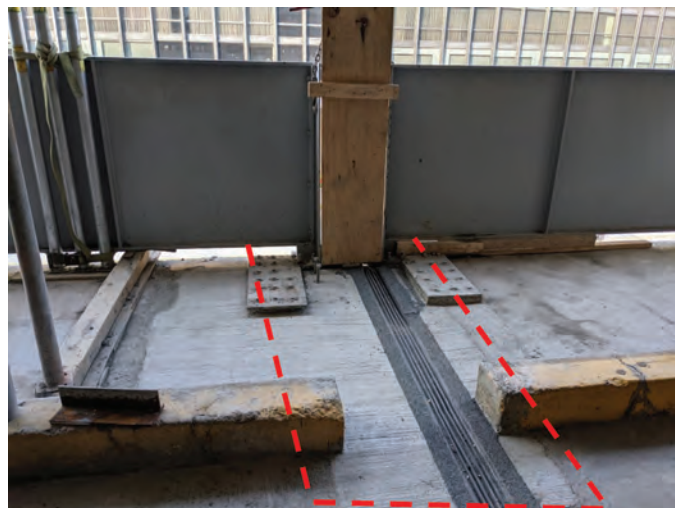
Fig. 6: Dropped infill block replaced with monolithic concrete (original position of infill block outlined)
