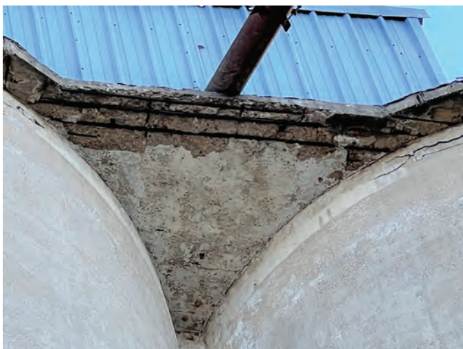
Deterioration at the silo overhangs
