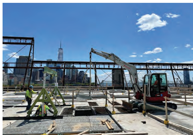
Installation of new precast plank
