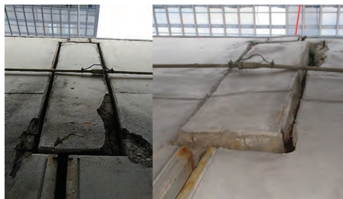
Fig. 5: Dropped, rotated, and spalling concrete at infill blocks
