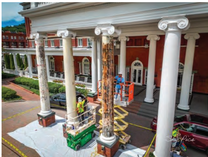
Restoration of the existing portico wood columns with FRP wrap and painting in progress
