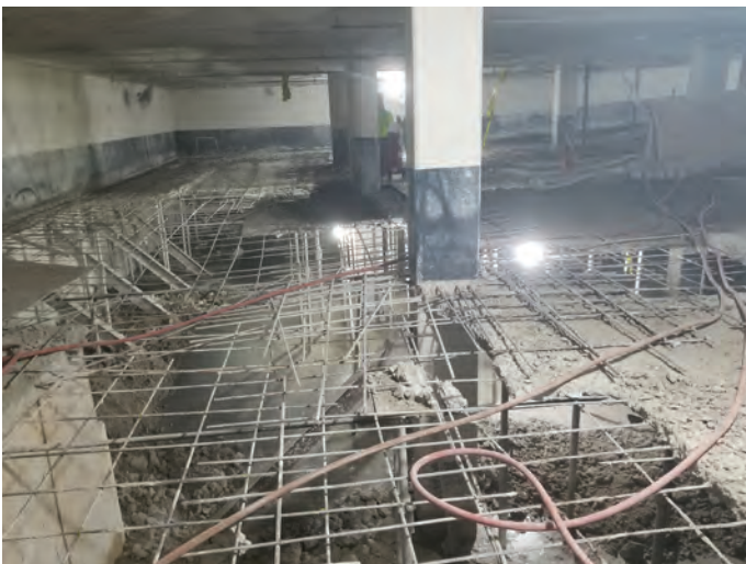
Fig. 6: Full depth slab repair areas in the garage
