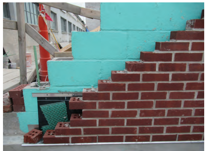
Fig. 9: South parapet reconstruction
