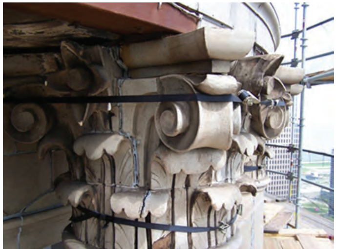
Fig. 1: Loose terra cotta secured with straps
