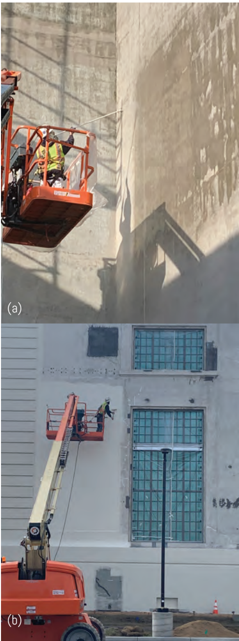
Fig. 6: Application of corrosion inhibiting coating, a) Application 1 and b) Application 2
