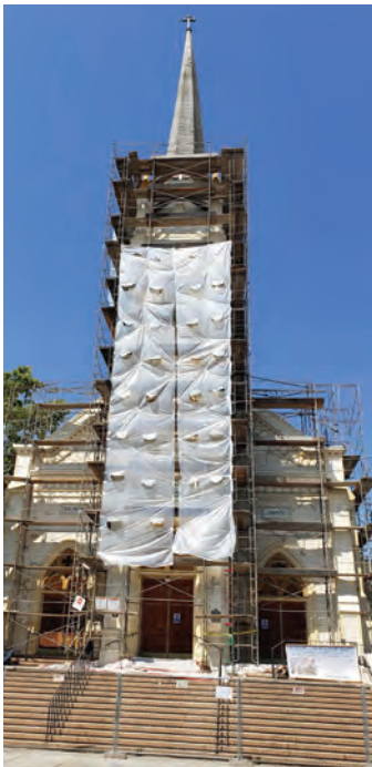
Fig. 4: Scaffolding erected with tarps to prevent overspray and direct sunlight
