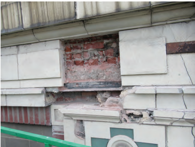
Fig. 6: Inspection opening at terra cotta water table
