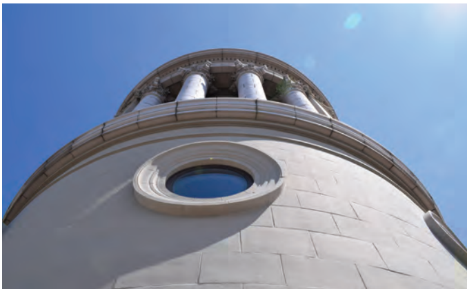
Fig. 4: Total of 32 fiberglass columns replaced in 2009 (photo in 2021)
