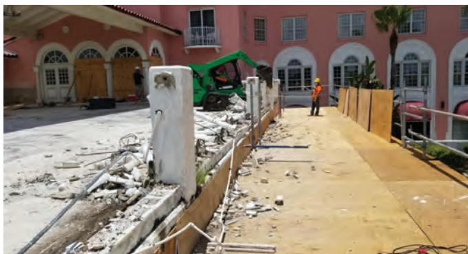
Fig. 4: Wide scaffolding installed over the road to serve as a working platform and debris control
