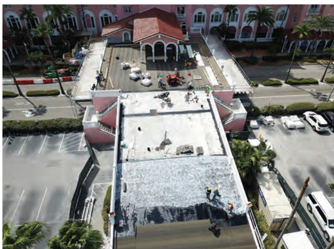
Fig. 5: Ariel view of completed structural repairs and waterproofing application on the bridge and ramp
