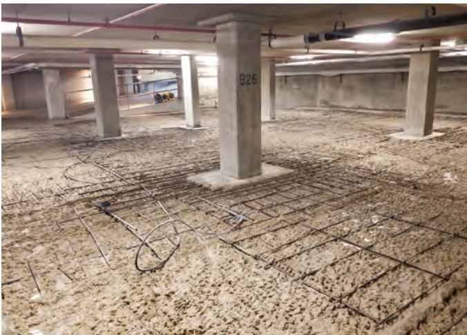
Fig. 5: Garage slab surface after hydrodemolition
