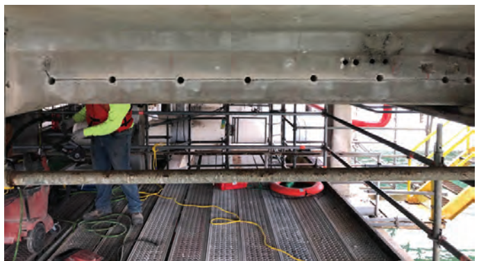
Fig. 4: Drilling anode holes
