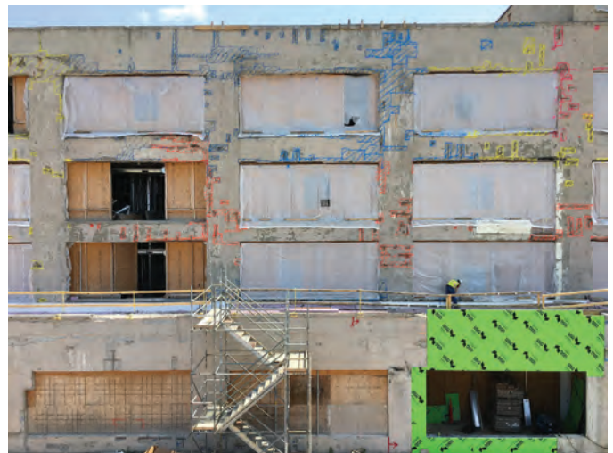
Fig. 8: Concrete repairs on west façade
