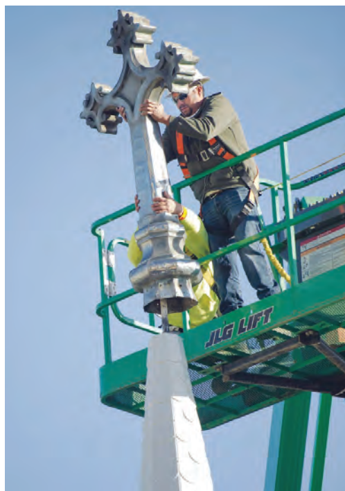
Fig. 3: New cross being installed to the steeple
