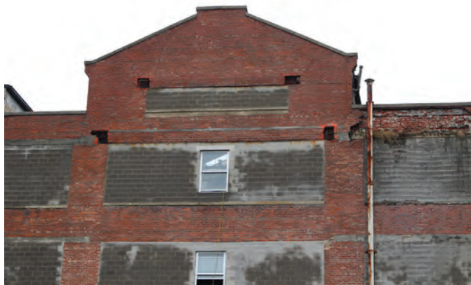
Fig. 3: Extensive concrete facade deterioration
