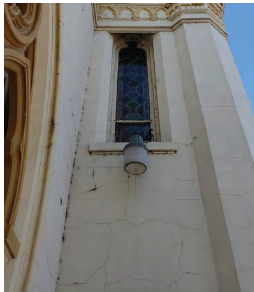
Fig. 2: Extensive cracking in the exterior plaster
