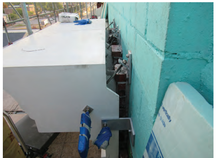
Fig. 13: Stainless steel anchors and hooks used to anchor the cornice to the reinforced concrete masonry backup wall
