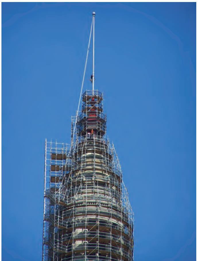
Fig. 2: Scaffolding around the entire 37th to 52nd floors allowed engineers to inspect every square foot of the façade
