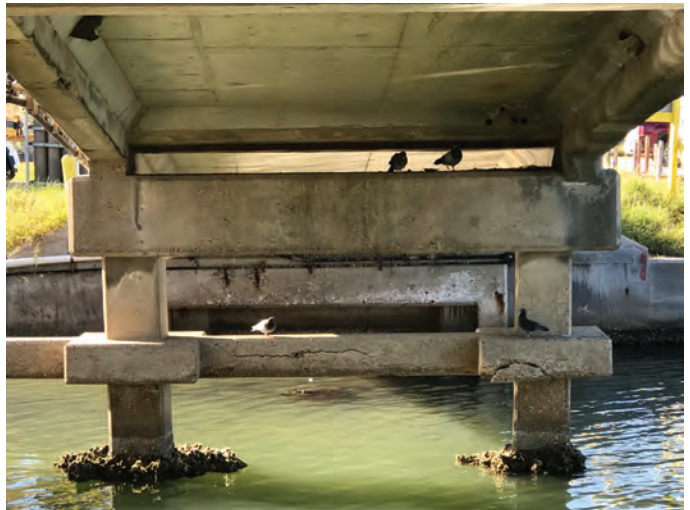
Fig. 3: Visible concrete deterioration
