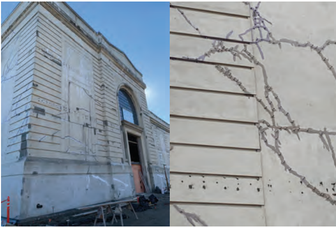
Fig. 5: Crack injection at exterior walls
