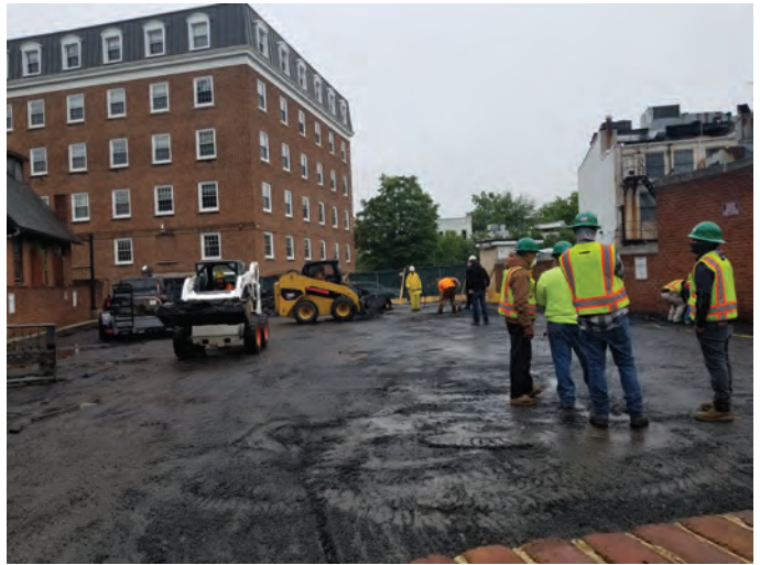
Fig. 1: Asphalt topping removal at surface lot
