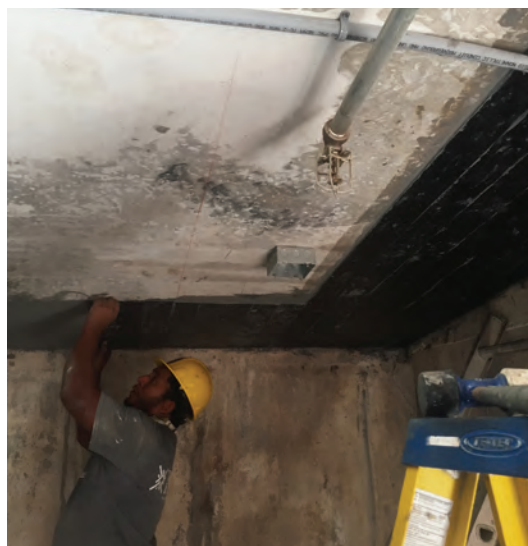
Fig. 3: Application of CFRP externally bonded strengthening below the existing repaired precast planks
