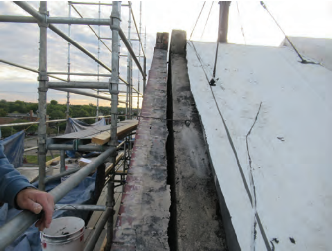
Fig. 5: Displacement of brick cladding on the north facade
