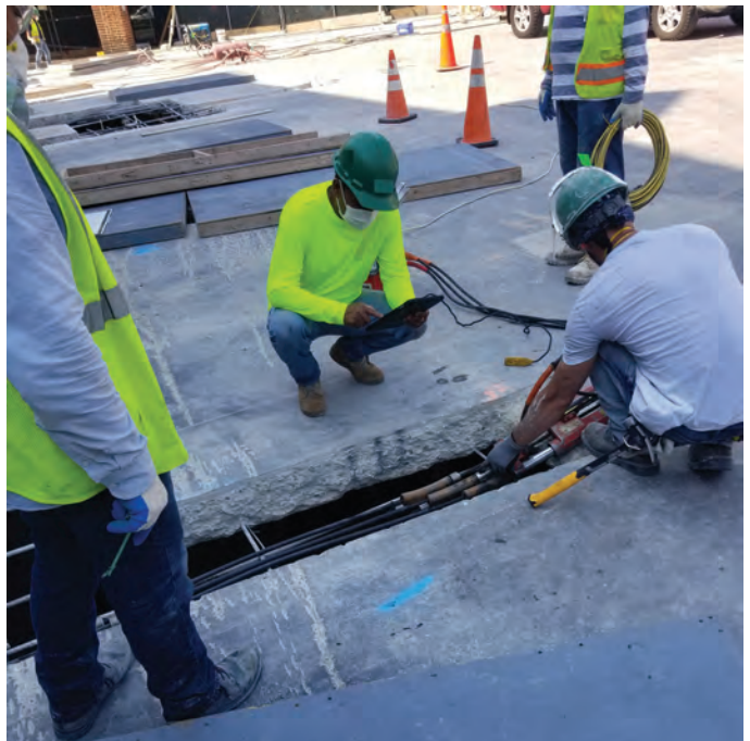
Fig. 2: Stressing repaired post tension tendon during structural slab repairs at surface lot
