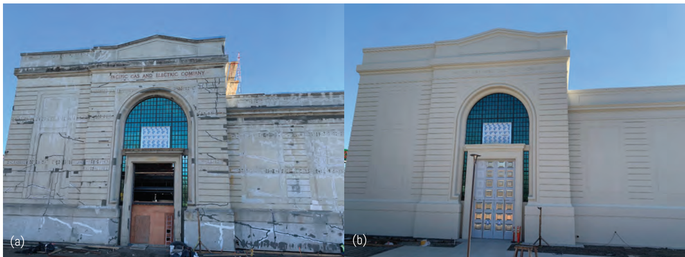
Fig. 7: Elastomeric protective coating: a) Before and b) After
