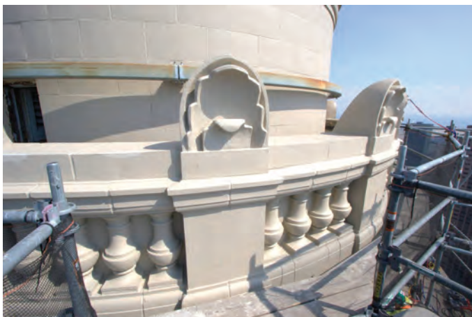
Fig. 5: Fiberglass-reinforced coating conformable and color-matched to salvagable terra cotta
