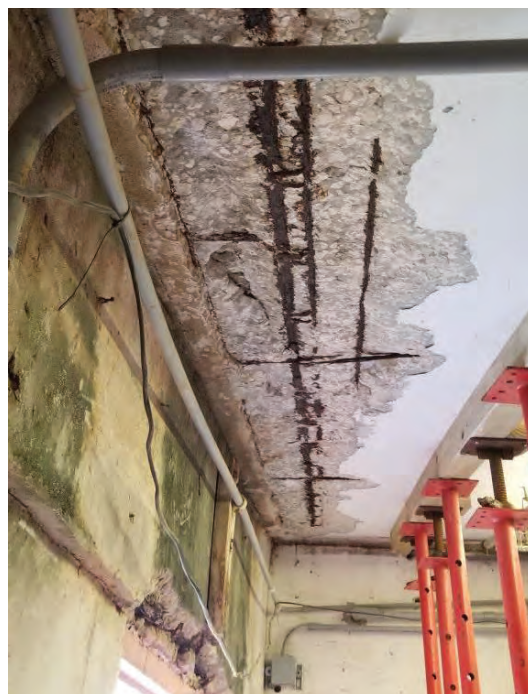
Fig. 2: Deteriorated precast prestressed ramp planks and spandrel beams at the elevated ramp structure with shoring
