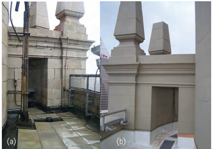
Fig. 6: Renovation of structurally failing balconies: a) Before renovation and b) After renovation
