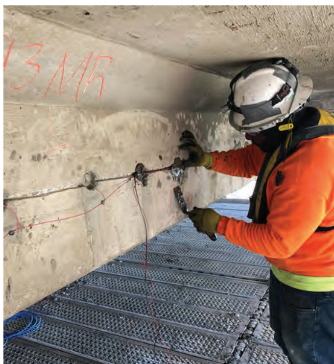
Fig. 6: Grouting in two-stage anodes
