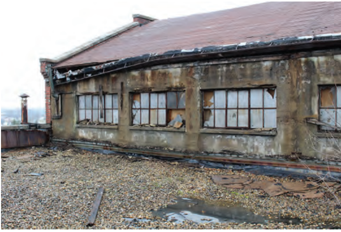
Fig. 4: Unstable and distressed areas on south facade
