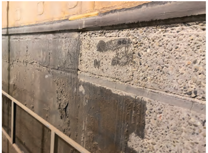
Fig. 3: Partially removed pre-existing coal tar coating
