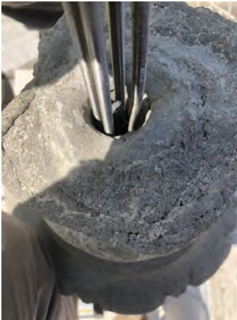
Fig. 5: Securing reinforcing bars
