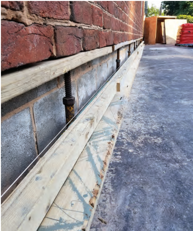
Fig. 4: Formwork for new curb to aid perimeter waterproofing at the surface lot
