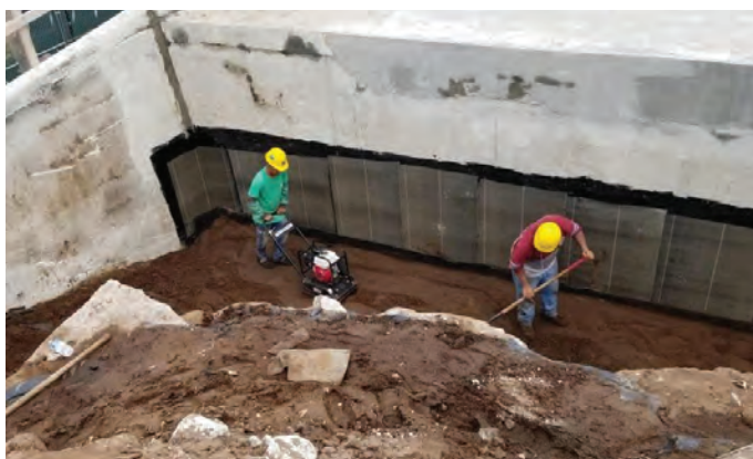
Fig. 6: Excavated area and waterproofing application on the rear foundation wall near the middle of the ramp
