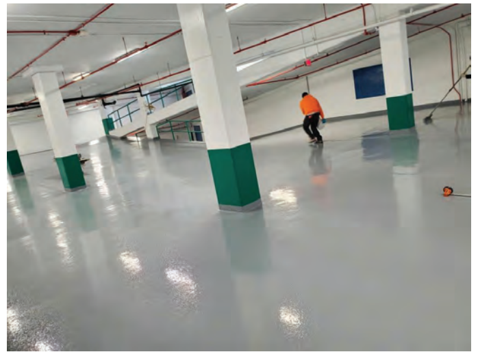
Fig. 7: Installation of topcoat for urethane traffic coating system in the garage
