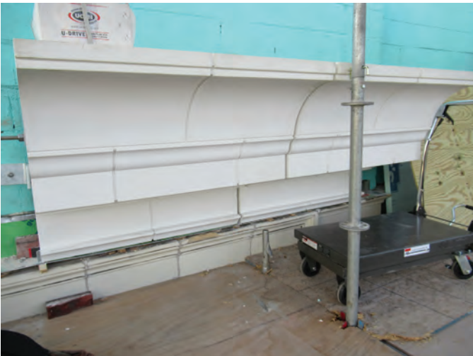
Fig. 12: Glass fiber reinforced concrete (GFRC) cornice replicating original terra cotta cornice units
