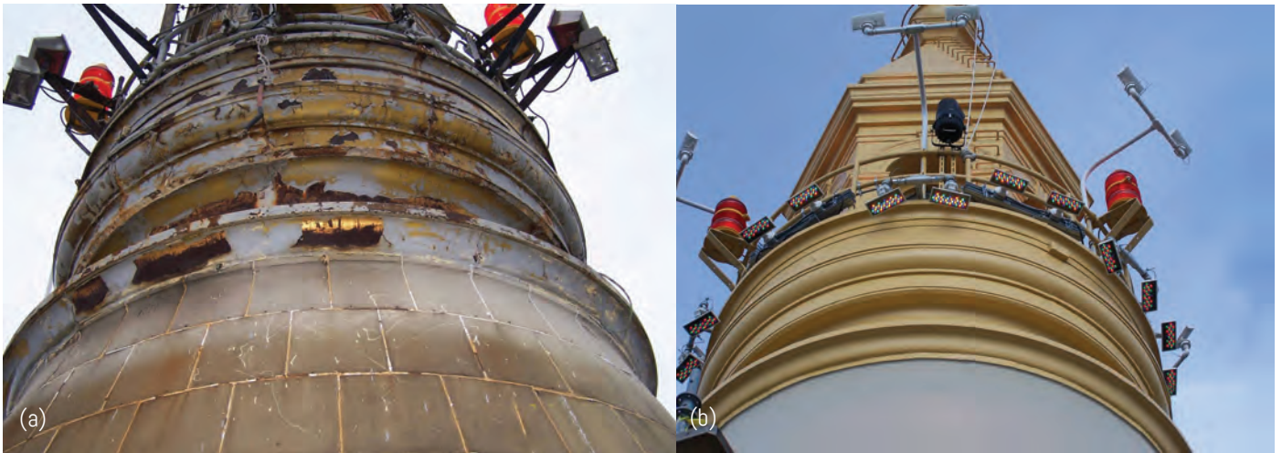
Fig. 3: a) Cracked and rusted cast iron cornices replaced with new steel duplicating shape of original, and b) Fiberglass reinforced polyurethane liquid applied membrane in custom gold to match original
