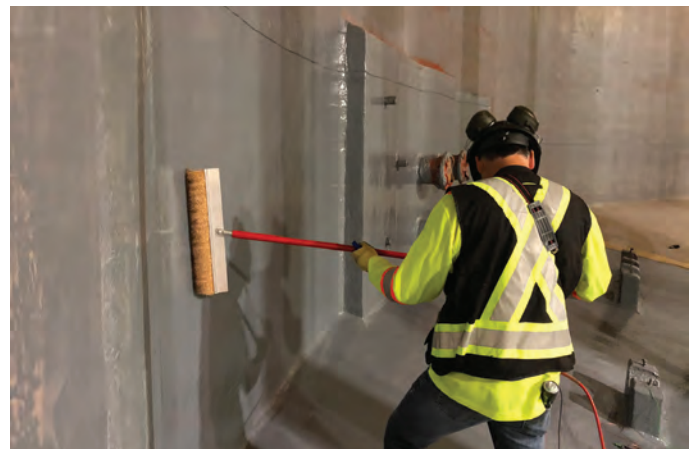
Fig. 7: Holiday/spark testing
