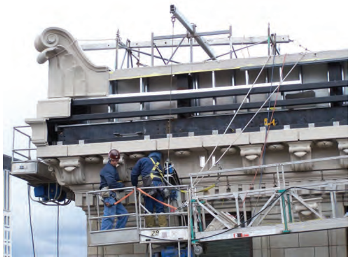
Fig. 7: Fiberglass units installed to new steel framing
