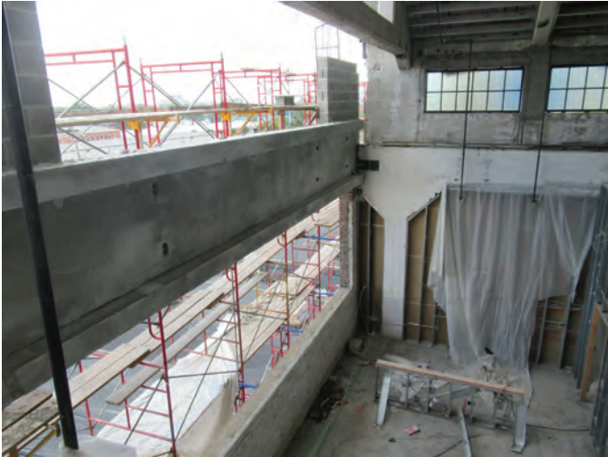
Fig. 10: Precast concrete girder set over window opening at south gable
