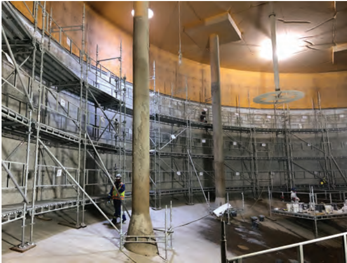
Fig. 4: Access scaffolding set up inside the digester
