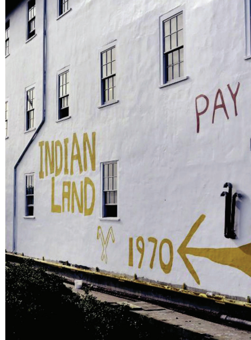
Fig. 12: New tracings of political statements on repaired concrete substrate
