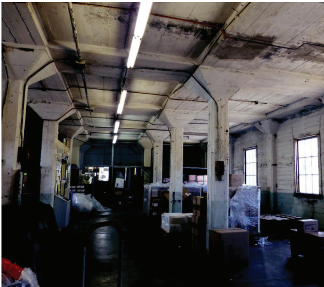
Fig. 7a: Interior area before restoration
