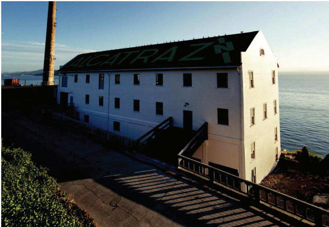
Fig. 13: View of Quartermaster Building after restoration the project to identify efficient and effective solutions to the planned repairs and unforeseen conditions
