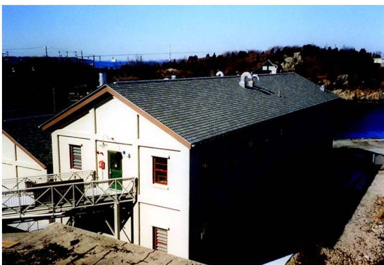
Before and after complete repair and protection system application
