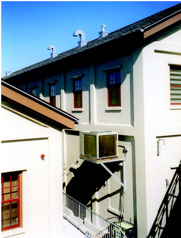
Before and after photo of repair of spalls and corner detail
