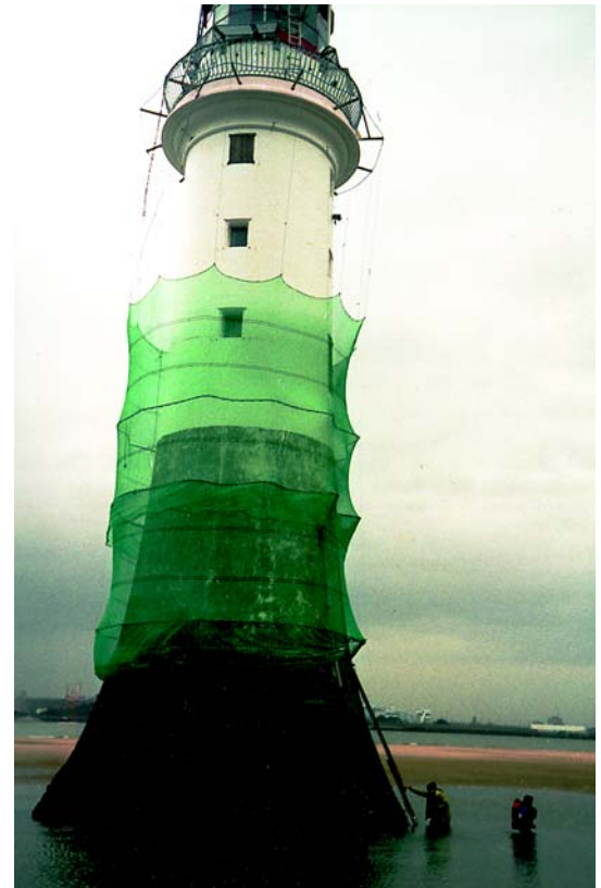
Figure 7: Containment net positioning
