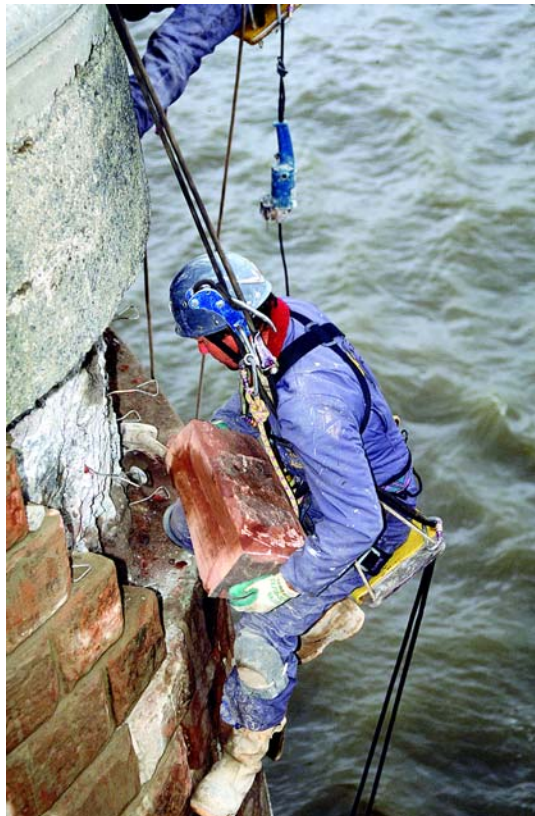
Figure 6: Rebuilding of the seawall
