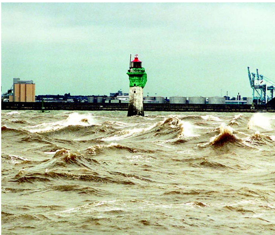
Figure 4: Project site at high tide
