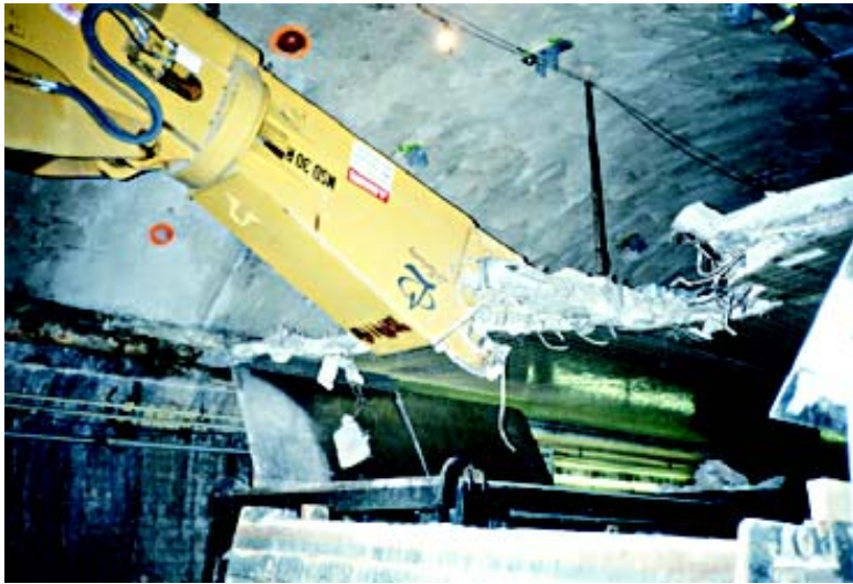
Fig. 3: Concrete demolition of the existing ceiling
