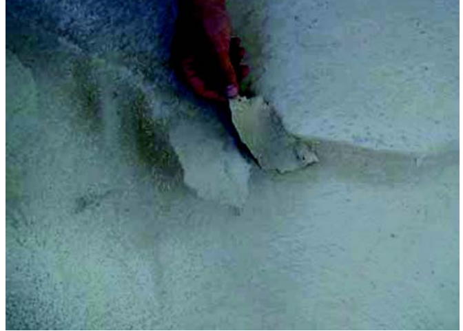
Polymer float condition also due to overwatering, improper mixing, or both, whereby polymer rises to the surface, displaying a soft, rubbery layer that is easily peeled away
