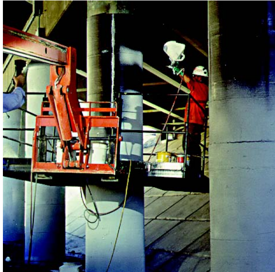
Spray application of acrylic coating for UV and abrasion protection
