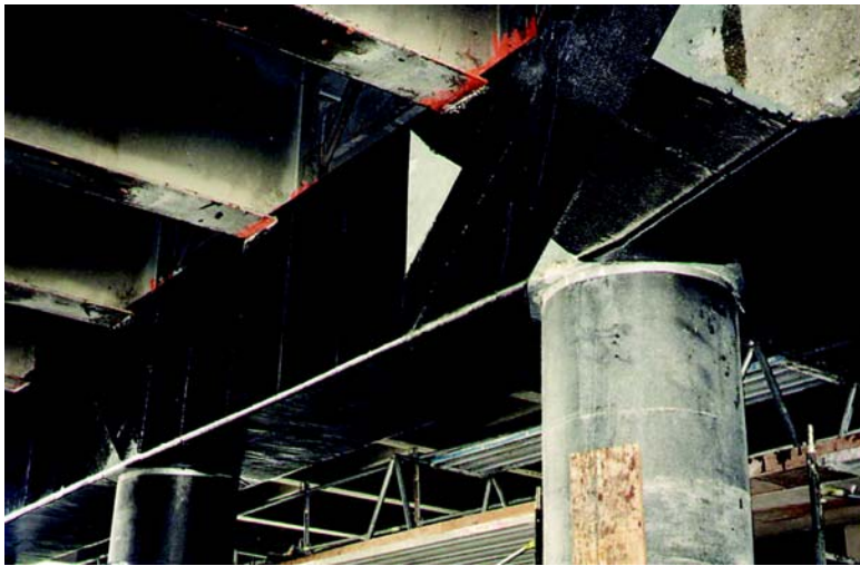
Bridge bent strengthening at State Street overpass
