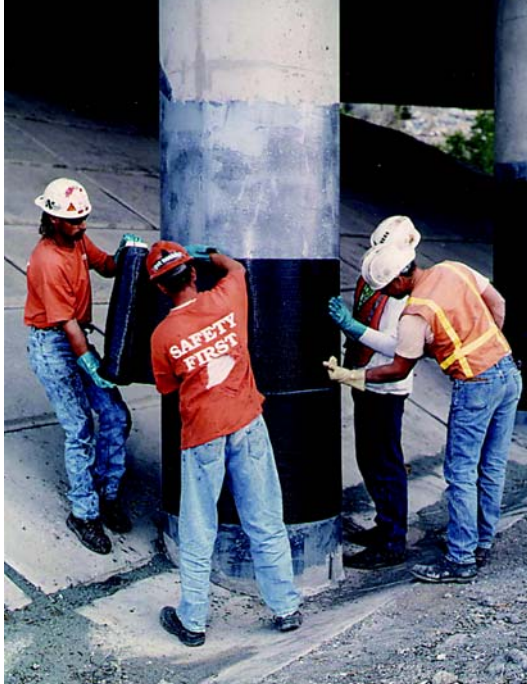
Wrapping bridge pier with carbon fiber fabric
