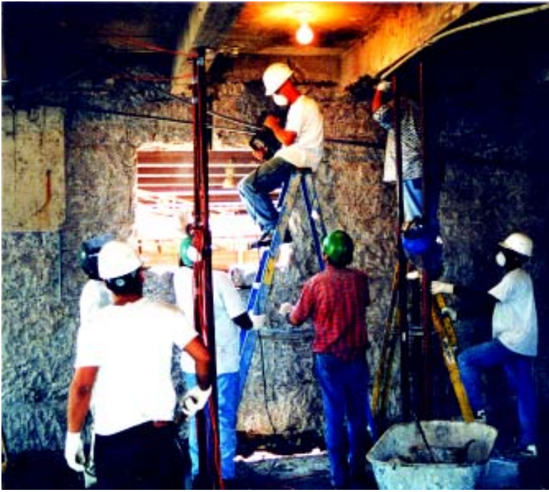
Figure 3: Workers remove deteriorated concrete
