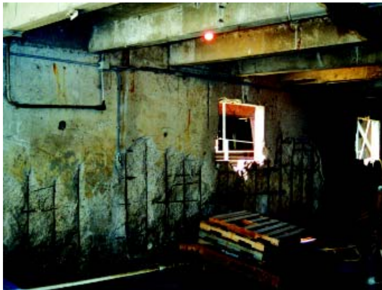
Figure 1: West wall (prior to start) on south end of room
