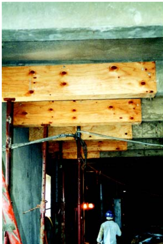
Figure 6: Wood box forms used for beam repairs
