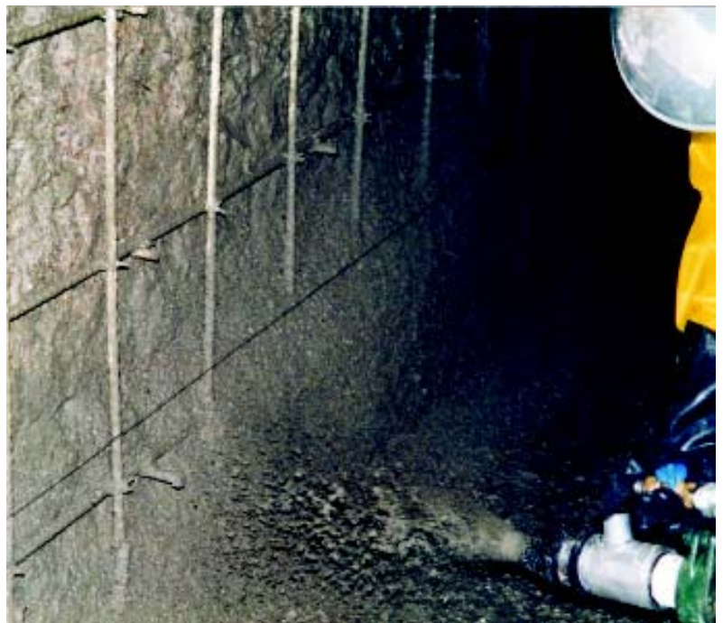
Figure 5: Shotcrete application
