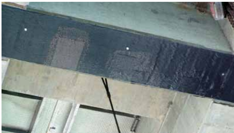
Fig. 1: Externally bonded FRP to a concrete beam
