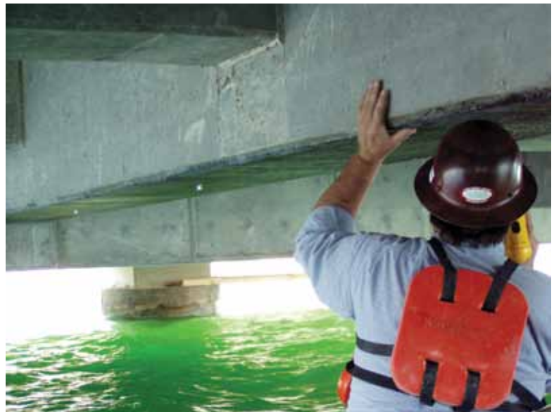
Fig. 3: Inspector examining the FRP concrete system
