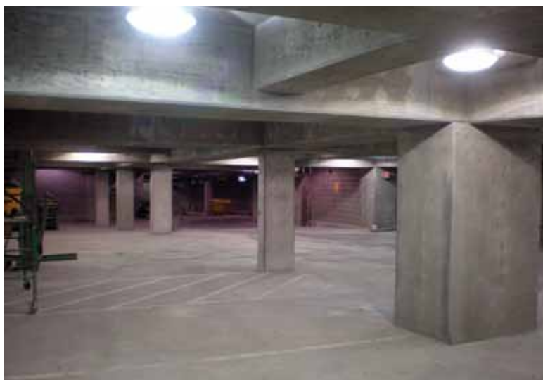
Finished beams and columns tied together
