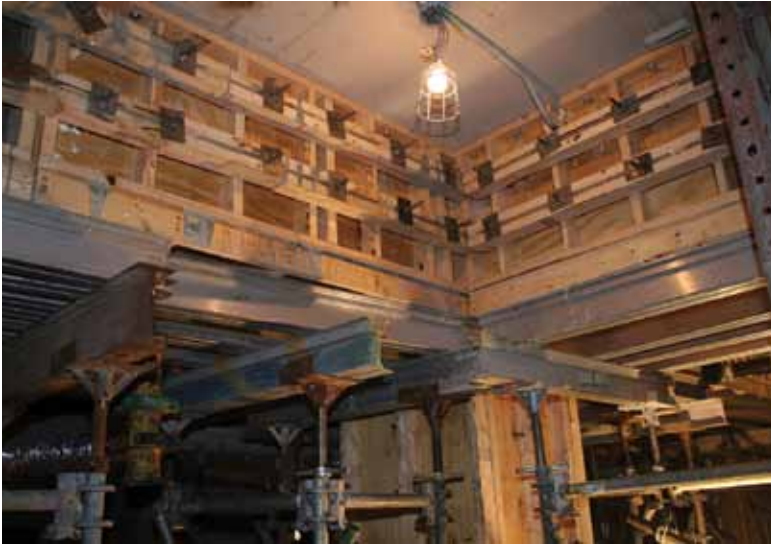
Example of typical formwork at the beam-column intersection
