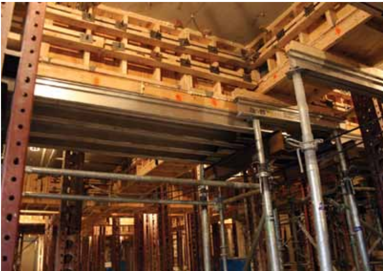
Structural shoring and formwork in place—this demonstrates the tight working area
