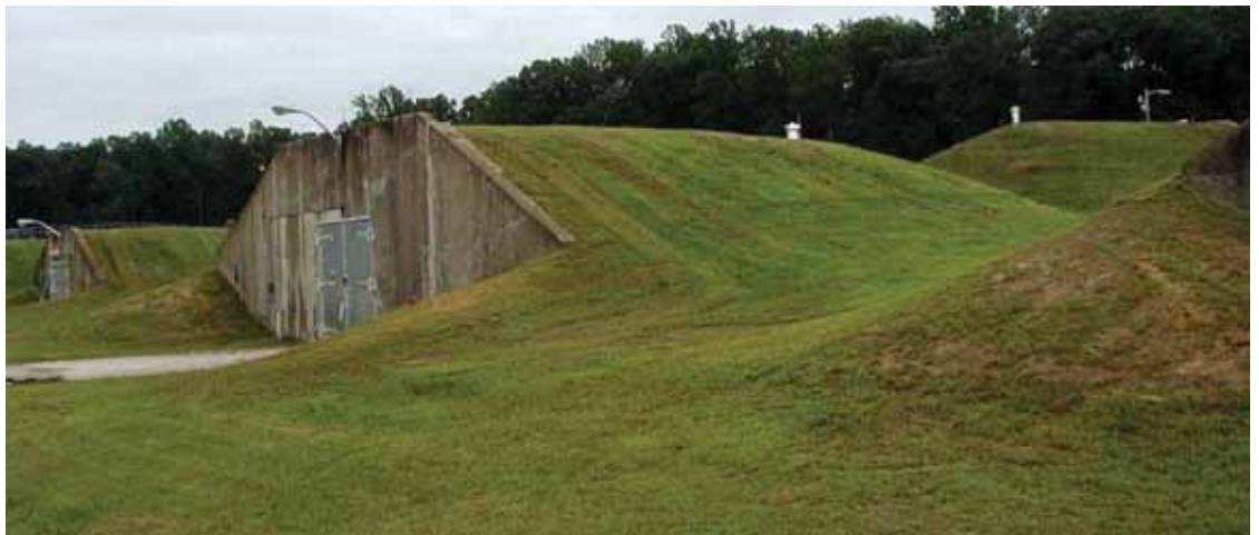
Typical steel arch earth-covered magazine (ECM)
