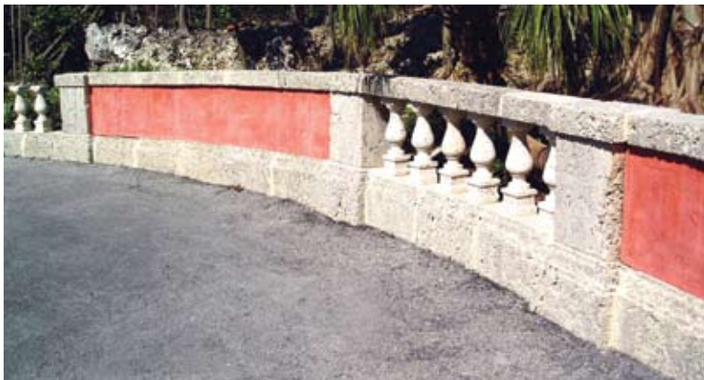
A balustrade reassembly in progress (left) and completed balustrade assembly (right)
