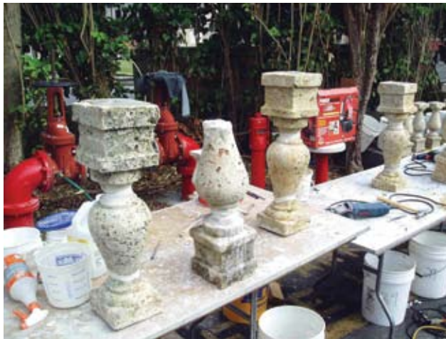
A newly cast replacement (left) and original centuries-old balustrade to be repaired
