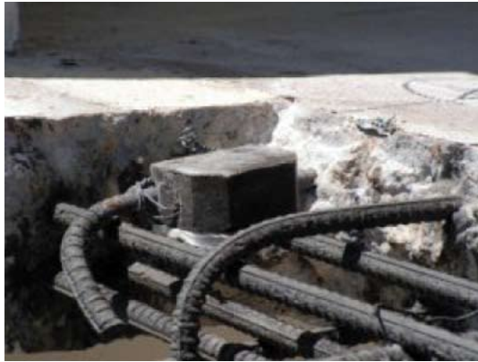
An embedded galvanic anode, with "V" notch easily attached to reinforcement before installation of repair mortar
