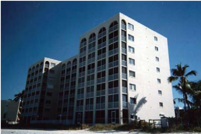
Completed balconies at rear elevation facing the Gulf of Mexico
