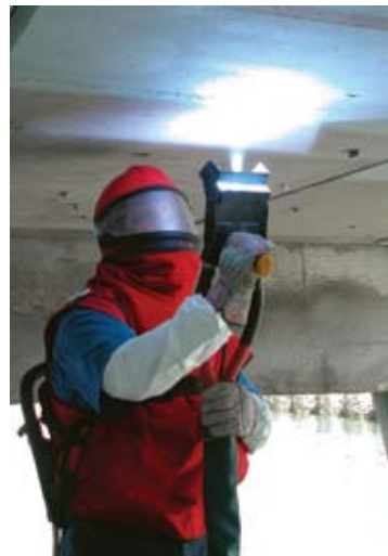
Application of activated arc sprayed zinc
