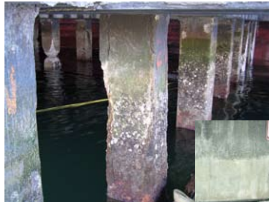
Typical pile before repair and galvanic jacket installation
