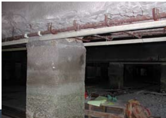
Activated distributed anode strips installed in pile cap
