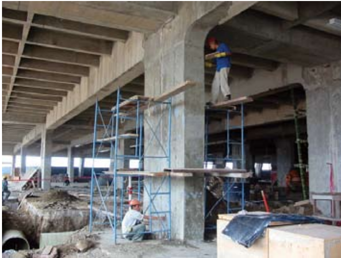
Fig. 4: Filling the gaps with a special high-strength, low-shrinkage rheoplastic repair mortar
