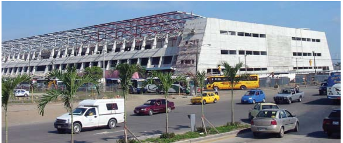
Fig. 1: Overall view of bus terminal
