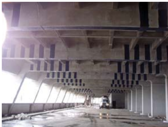
Fig. 6: Wrapping of the overhead ramp support beams
