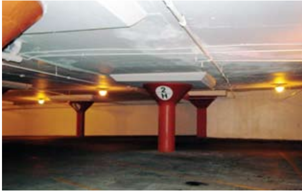
Garage, Level 2, following concrete repairs and painting
