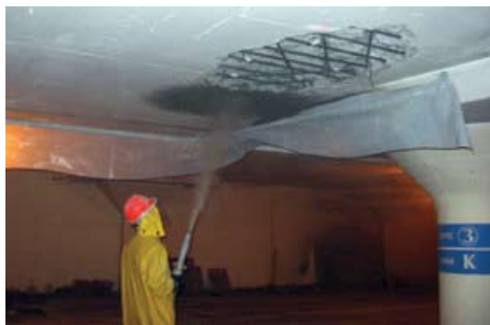
Shotcreting a soffit
