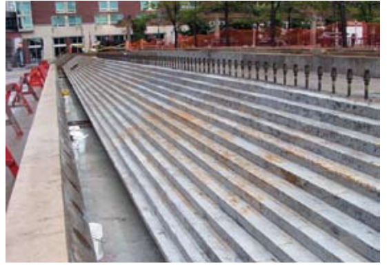
Water feature repairs underway
