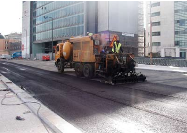
Application of cold asphalt
