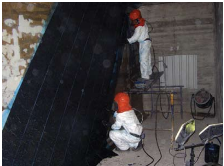
Internal reinforcement with CRFP fabrics
