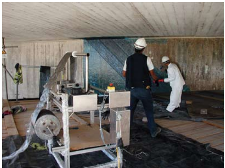
External reinforcement with CRFP fabrics
